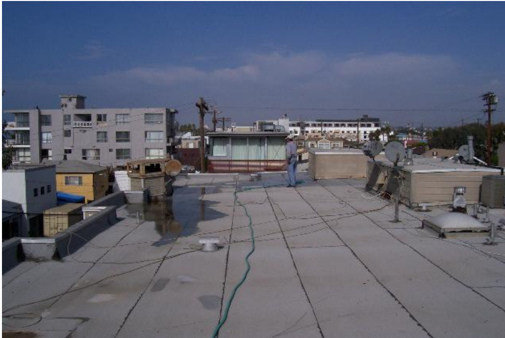
PF 01.133 PF 01- 133.jpg Roof: General shot.
